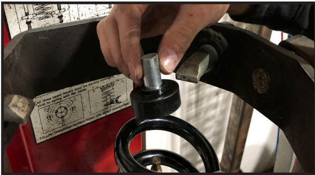
15. install bushing and sleeve onto the shock stud so its on top of the washer.
