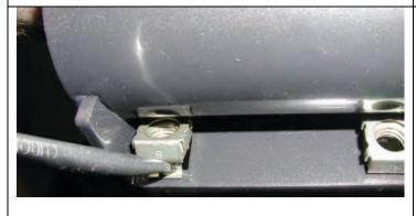
3. Remove light panel from frame assembly, it is held on by cable ties for transport only. Insert M10 caged nuts to inside of mount brackets on frame assembly, 4 places per bracket as shown.
