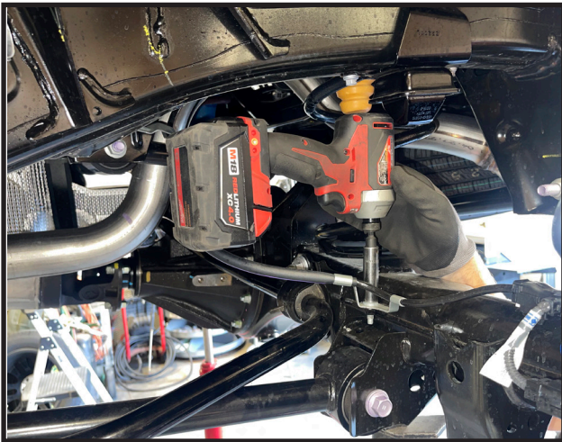
30. Carefully lower the rear axle down enough that the OE rear coil springs can be removed.
